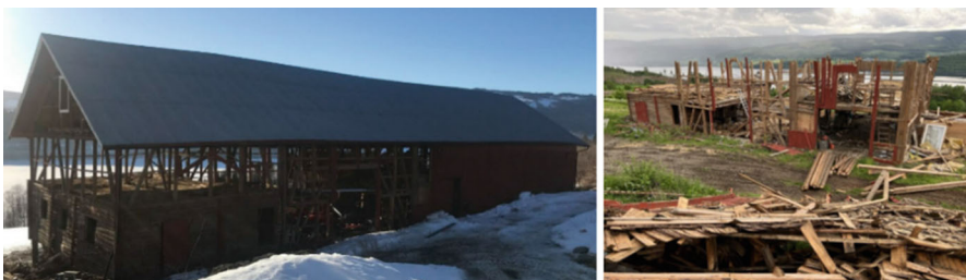
Fig. 1 Demounting the barn in 2022, provided by Omtre
