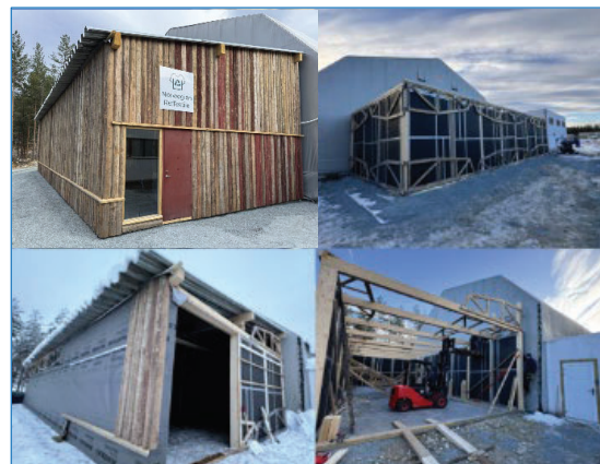
Figure 1: Pilot building for textile sorting. Reuse of glulam, nailplate-frames, barnwood and planks.
